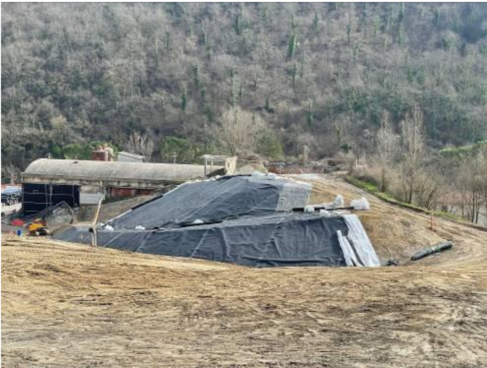
FIGURA 9: POSA TELI CAPPING IN AREA 2 SUD
