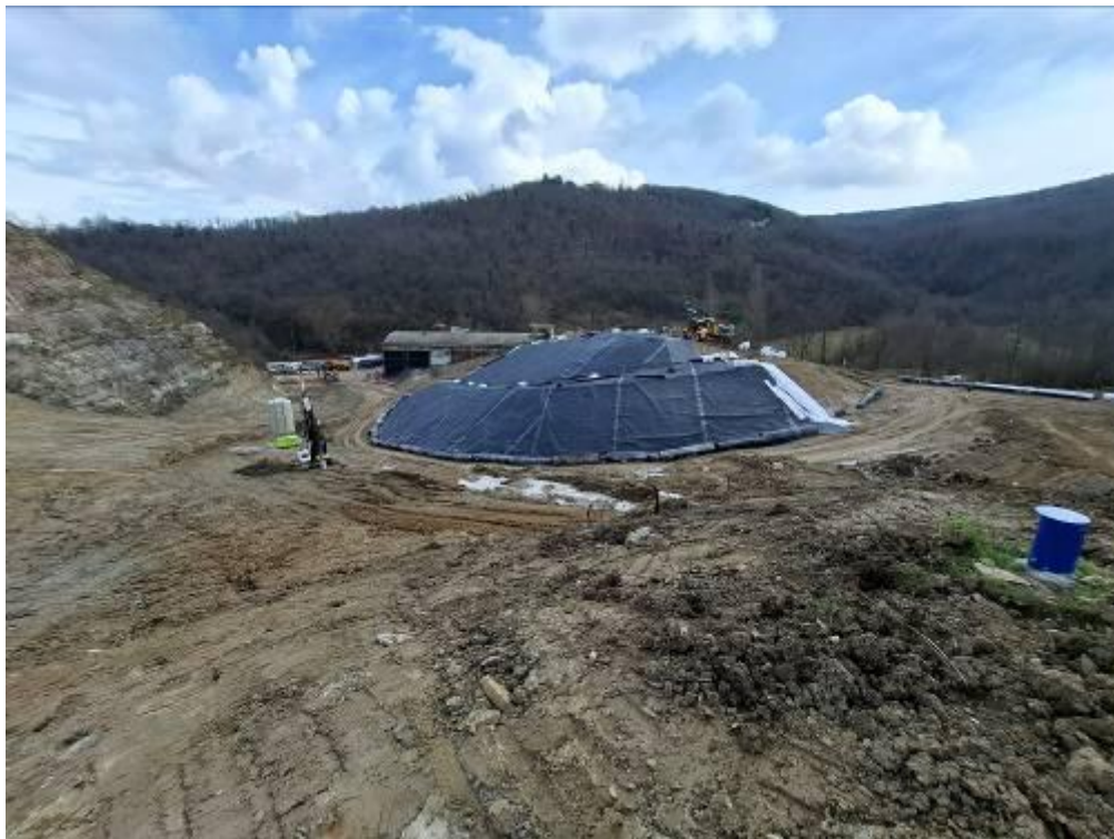
FIGURA 10: POSA TELI CAPPING IN AREA 2 SUD
